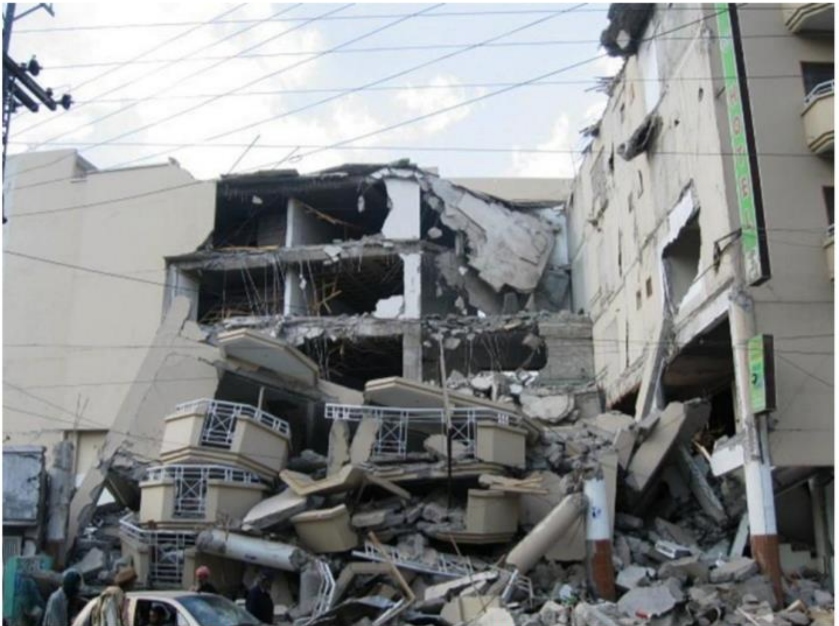
Figure 6: Collapsed Sangam Hotel building (in Muzaffarabad).
